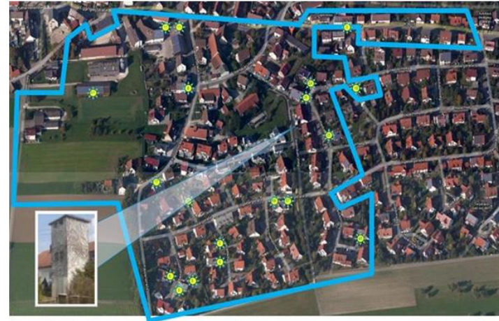
Test Area in Ulm, Germany (Overlaid of the roof solar potential analysis and the position of the PV systems and transformer station)
