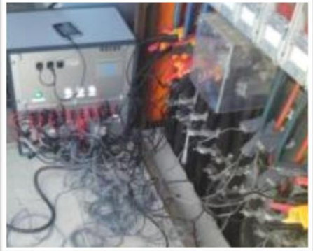
Measurement at 8 Transformer-feeders in second resolution
