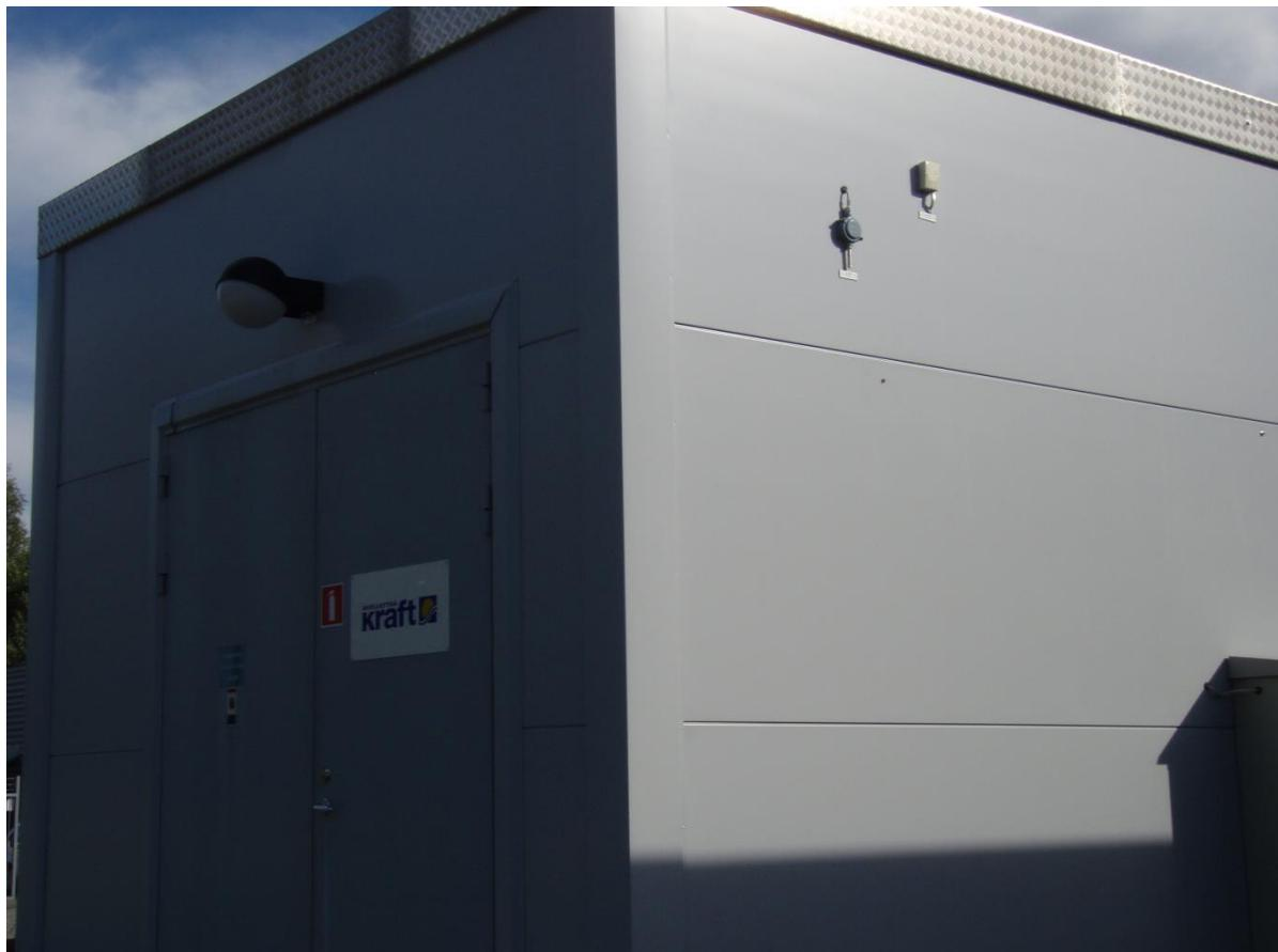
**Fig. 4-9: Photograph of temperature measurement devices at the H21 substation. Photograph was taken by SKR.**
