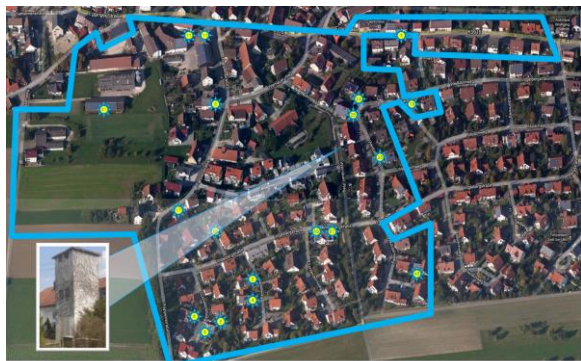
Airborne image of the test area Einsingen in Ulm (Germany) with the position of the PV systems (sun symbol) and the transformer.
