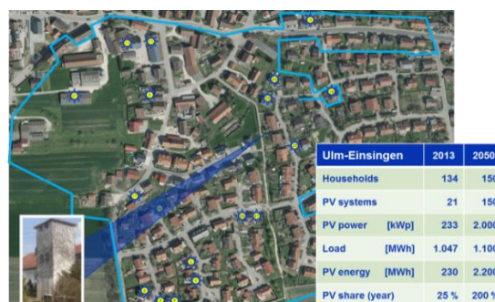
Fig 3. Airborne image of the Test area in Eisingen in Ulm, Germany, with the position of the PV systems and the transformer (source: HS Ulm)
